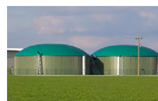
Installations de biogaz
